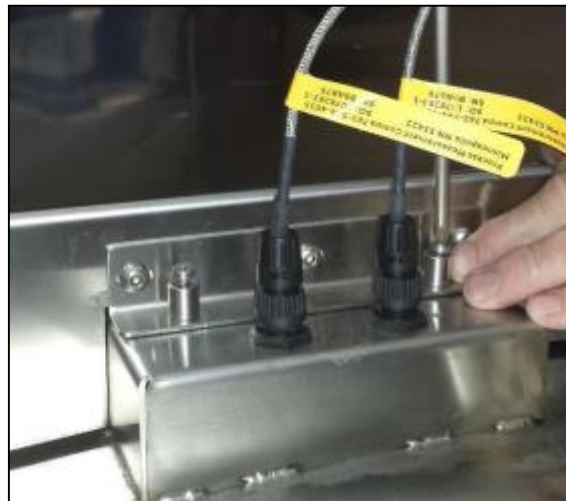
Figure 13 - Phillips Head Screws to Remove
